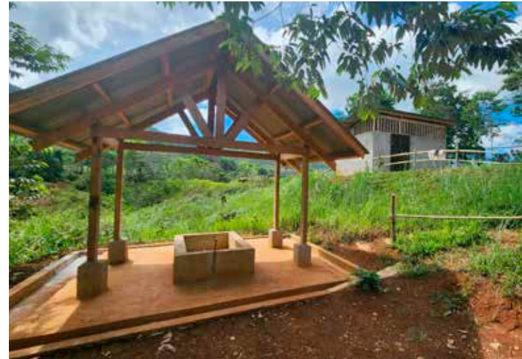
Newly constructed toilets and tubs at APC Mindagulos School. Mindanao, Philippines
